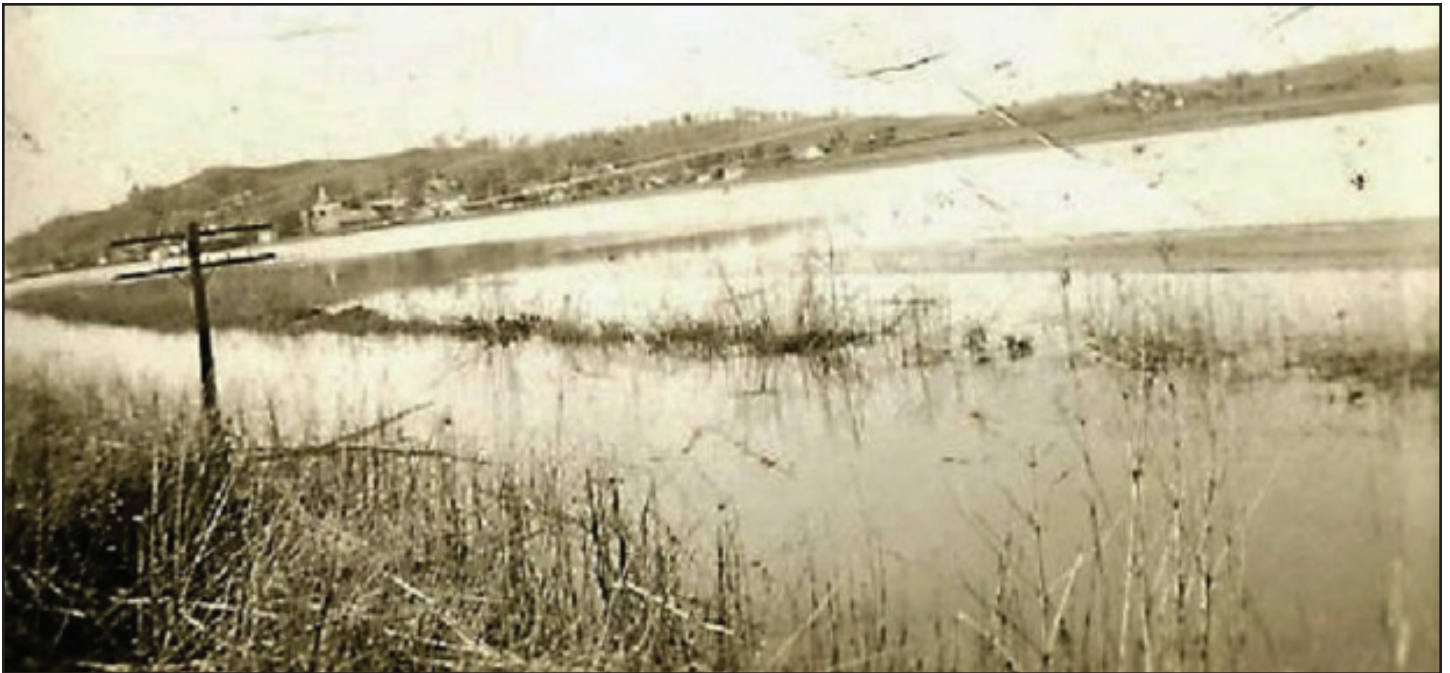
Flood water covers 45 highway south of Farley. Circa 1945.
